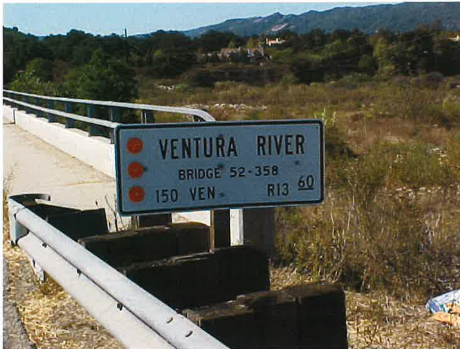
Baldwin Bridge on Ventura River (HWY 150)
