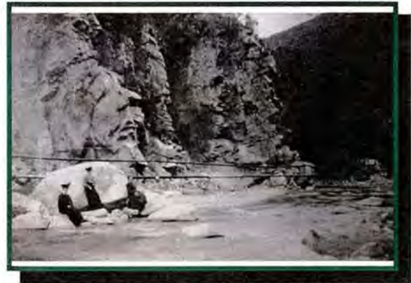
Photo 5 - Upstream Matilija Dam-site (early 1900s)
