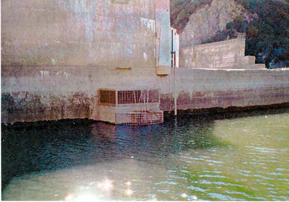
Existing outlet works intake.
