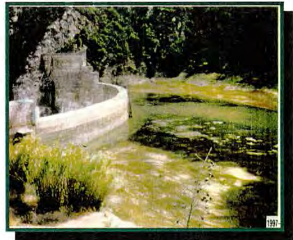
Photo 2 - Accumulated Sediment Behind Matilija Dam
