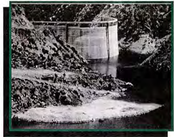
Photo 1 - View Upstream of Matilija Dam and Reservoir After Completion in 1947
